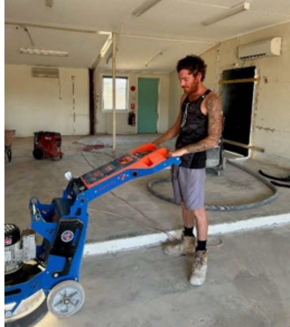
Work underway on renovating Burwarri.
