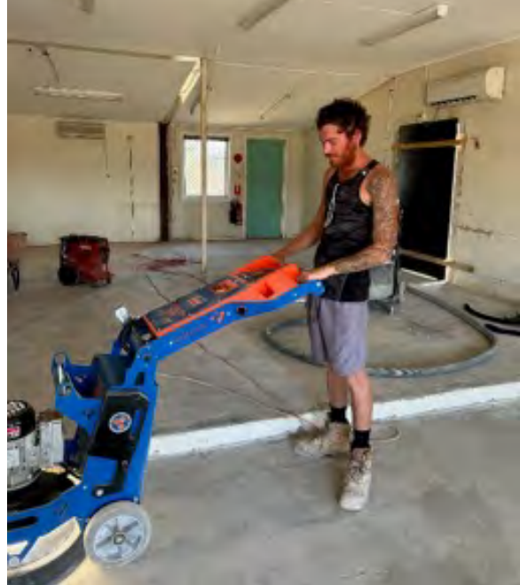
Work underway on renovating Burwarri.
